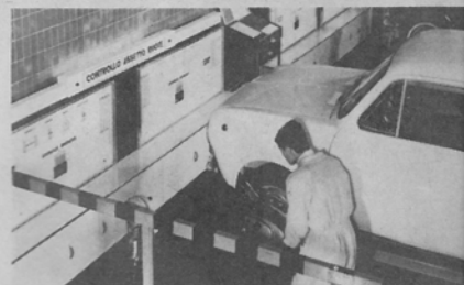
FRONT-WHEEL ALIGNMENT of camber, caster, toe-in is done at one of several stations along the line
