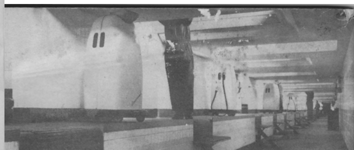
WORKING FROM BELOW, mechanics find the grease pit approach well-organized, safe and efficient
